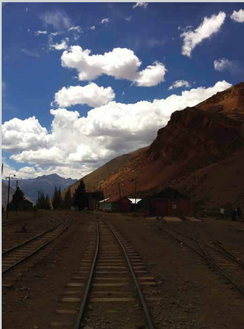
Abandoned railroad Photo credit: Fabien Fivaz
