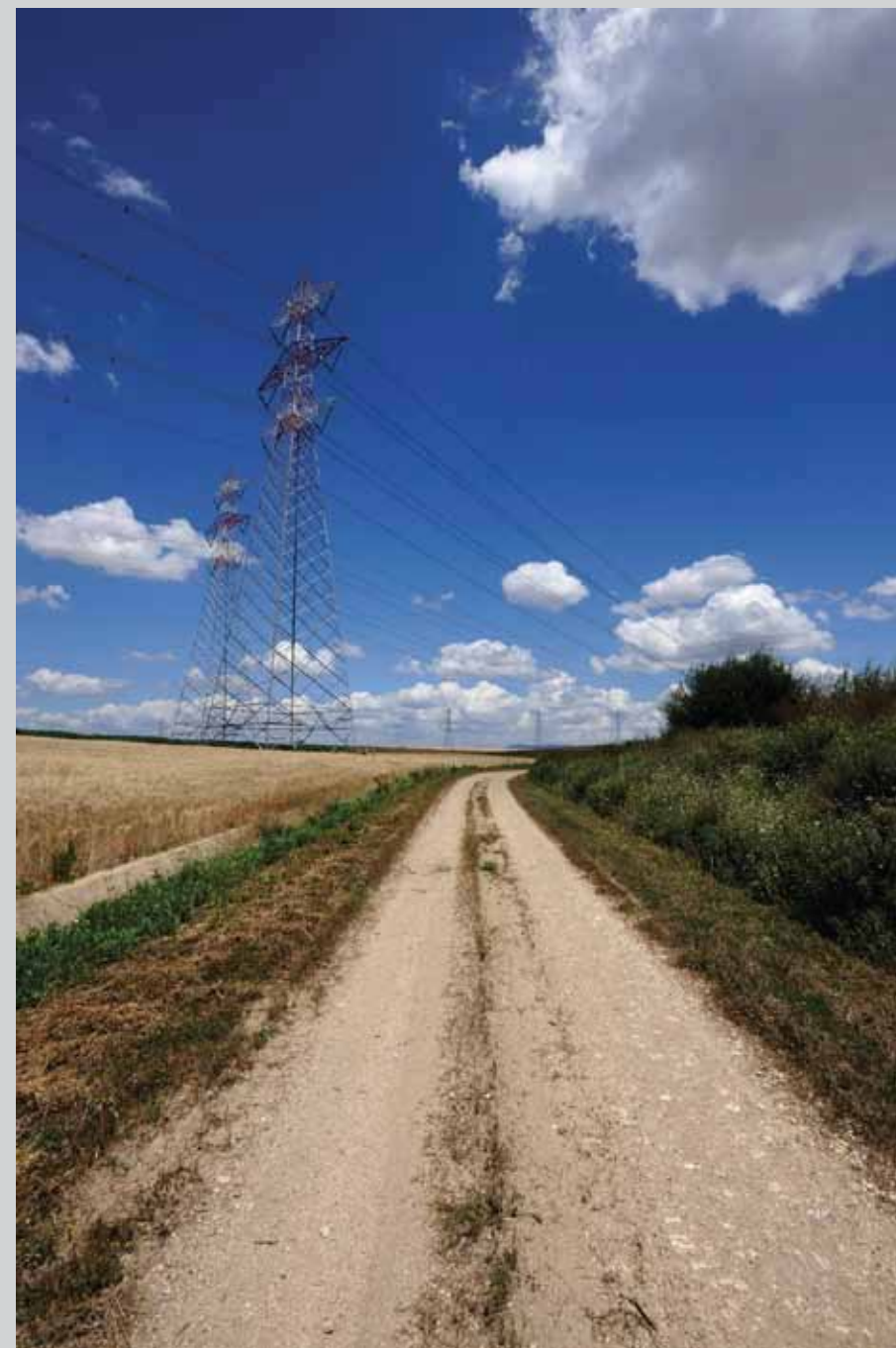
Transmission line adjacent to road
