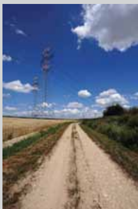
Transmission line parallel to existing transmission line
