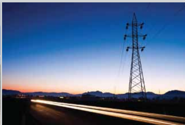
Transmission line adjacent to road
