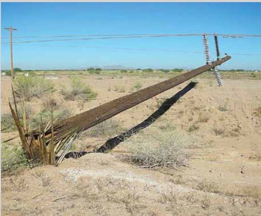
Transmission line storm damage Credit: Western Area Power Administration FY2011 Ten Year Capital Program PowerPoint
